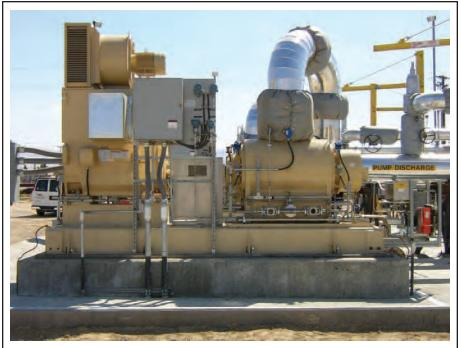
Multiphase pumping offers the unique ability to boost both gas and liquids in a single process with a single piece of machinery in both onshore and offshore applications. Shown here is a typical multiphase pumping unit in on onshore installation.
