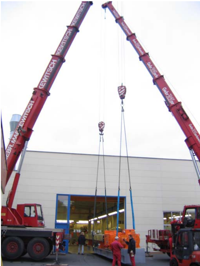
Loading of the twelve meter long ZSE 135 MAXX extruder.
