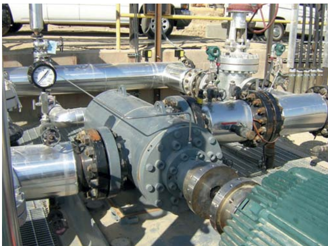
An increasing number of screw pumps are being used to transport stored oil products (photos: Leistritz Pumps)
