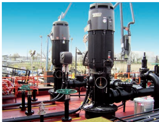
Top picture: Vertical "in-tank installation" of L5NT-Pumps Right picture: Pump and assembly
