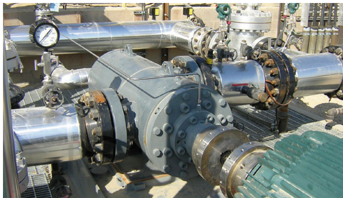
Fig. 4: Crude Transfer Pump
