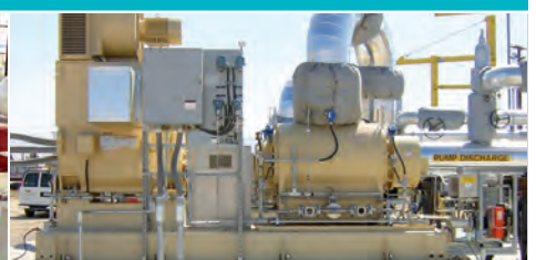
Leistritz Multiphase Pump with Insulation on a Californian Oil Field
