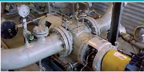
Leistritz Multiphase Pump on a Canadian Oil Field
