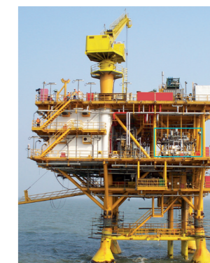
Offshore platform with a Leistritz multiphase pump
