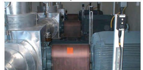
5 Crude Stripping Pump L4NG
