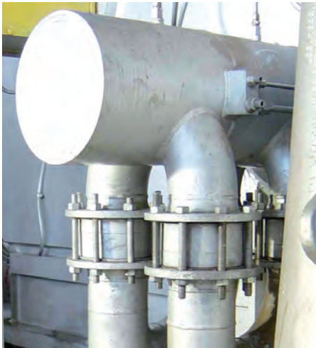
3 Reduction Gear Lube Oil Pump L3MG
