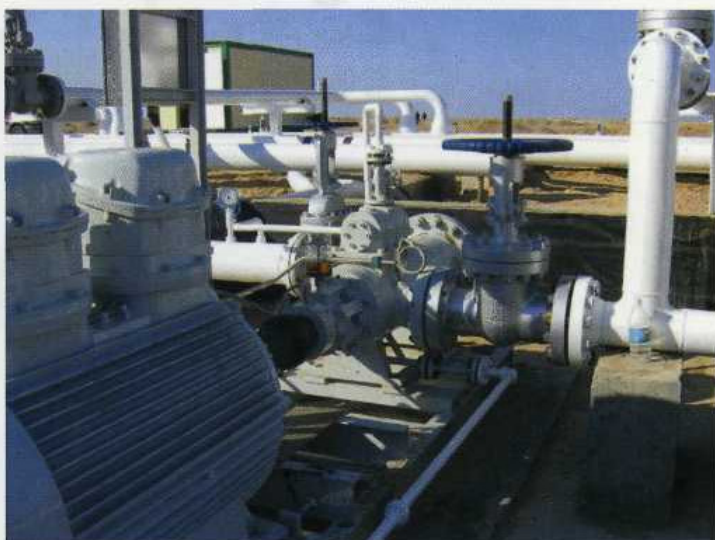
Leistritz three-rotor screw pump with 55 bar \Delta p as pipeline pump in Egypt
