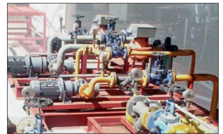
1 2 LO Transfer and Separator Supply Pump L3NG
