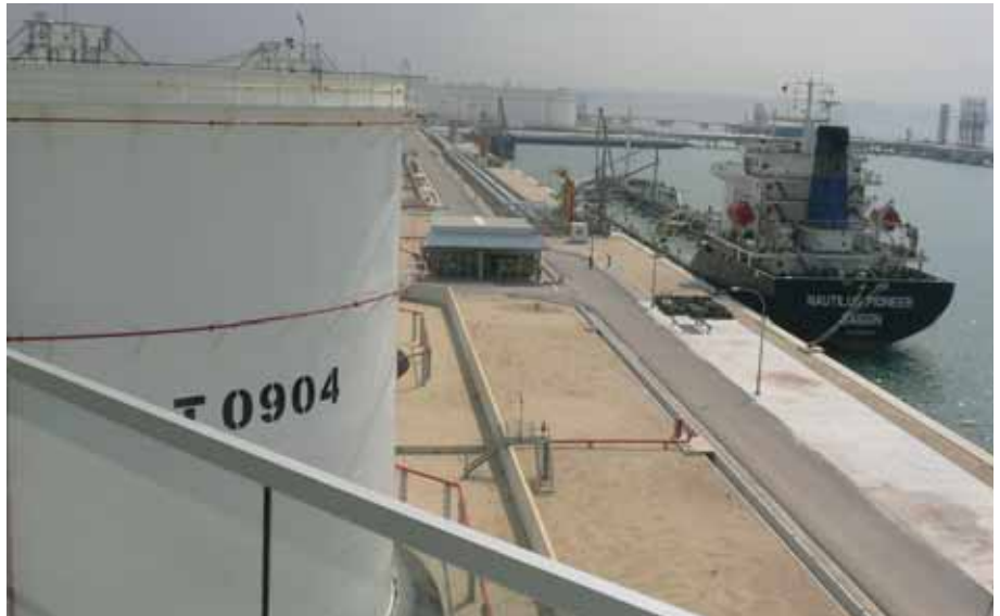
Storage and Loading Facility in Singapore
