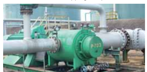
6 Leistritz HFO Transfer Pump L4MG
