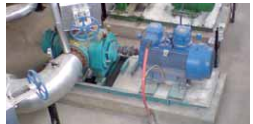
5 Leistritz Crude Oil Stripping Pump L4MG
